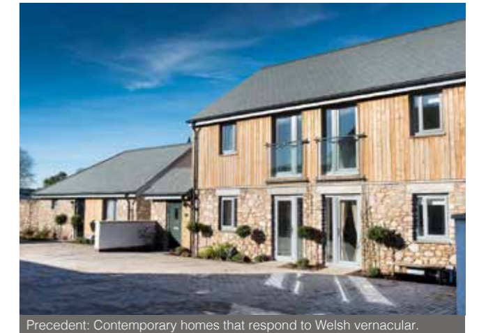
Precedent: Contemporary homes that respond to Welsh vernacular.
