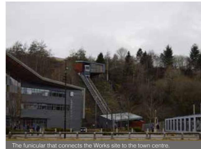
The funicular that connects the Works site to the town centre.
